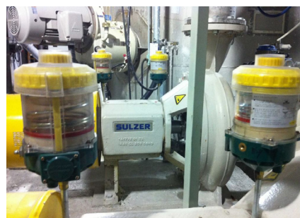
View of installation
